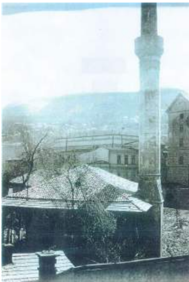
Sl. 21 Slikano sa sjeverozapada, trijem i minaret; u pozadini krov Narodnog pozorišta i Brdo džamija Fig. 21 Photographed from the north-west, portico and minaret; in the background, the roof of the National Theatre and Brdo Mosque
