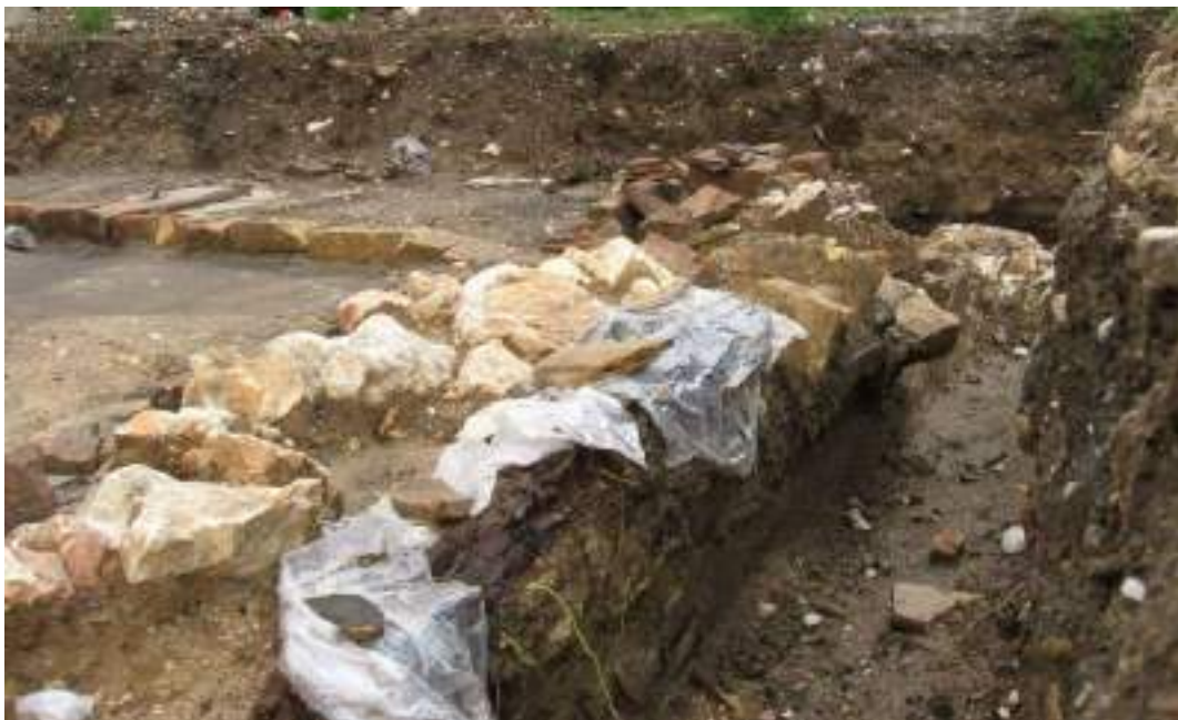
Sl. 14 Zid A mekteba, unutrašnja strana s ostacima grede i malternom oblogom pri dnu Fig. 14 Wall A of the mekteb, inner side with remains of beam and plaster near the base
