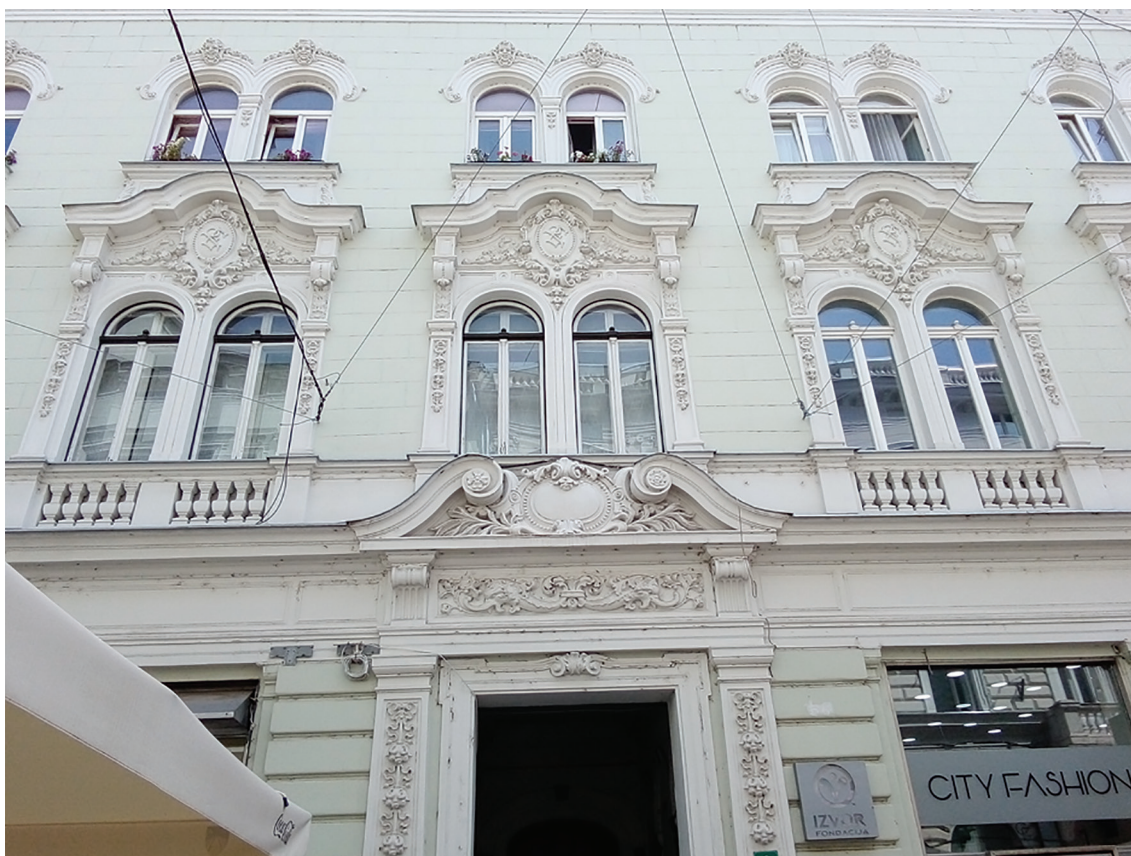
Slika 6. Pročelje zgrade porodice Pleyel Image 6. Façade of the Pleyel family's building
